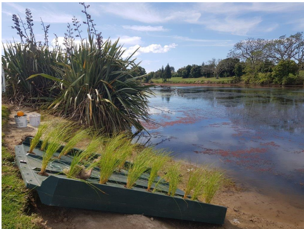
Figure 4.6: An AST style floating wetland being deployed in Awatapu Lagoon in 2019.
