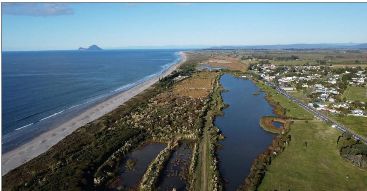
Figure 3.9: Western Matatā Lagoon (facing east) showing extensive cover of pampas grass with white flower heads in the sedimentation bay, western end of floodway bay 3, embankment separating the floodway bay 3 and 4, and along the edge of the walk way (May 2024).
